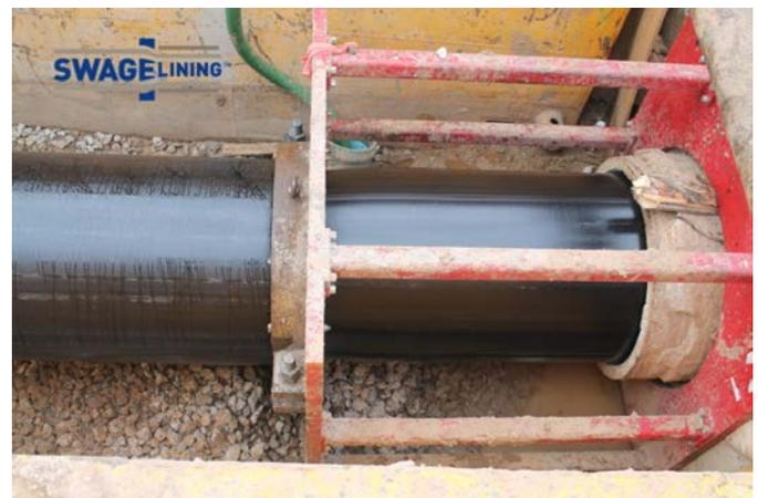
**During the Swagelining™ process the HDPE pipe is temporarily reduced as it is pulled through the reduction die.**
